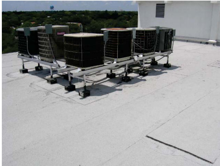
Asphalt Rolled Roof Covering
