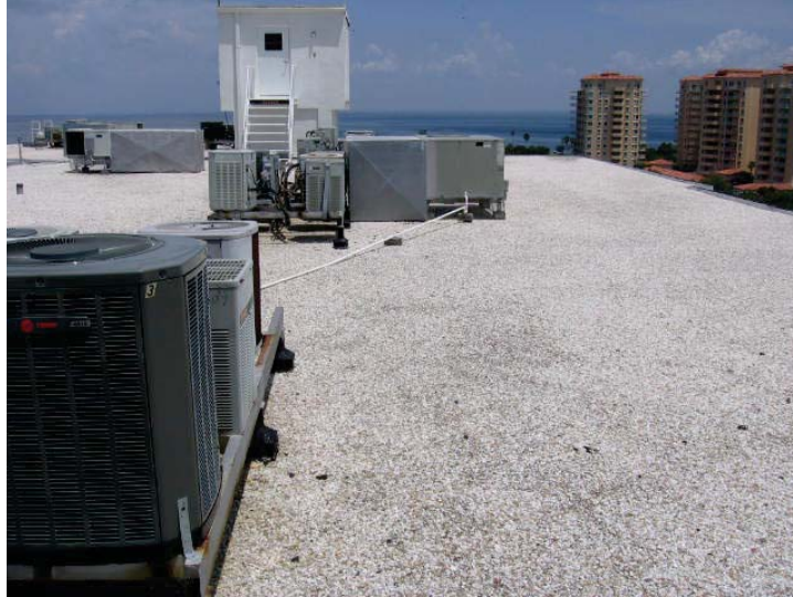
Tar & Gravel Roof Covering
